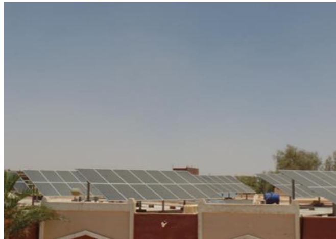
Figure 3. The 28 kWp Grid-connected PV system [12].
