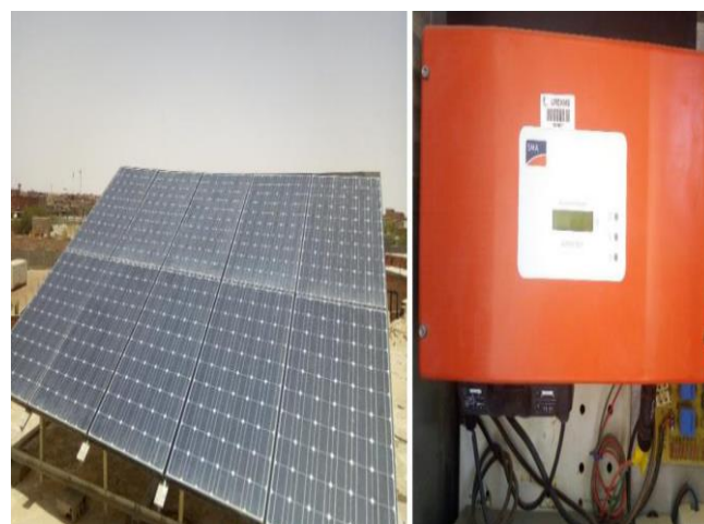
Figure 4. The 2.5 kWp PV system [14].
